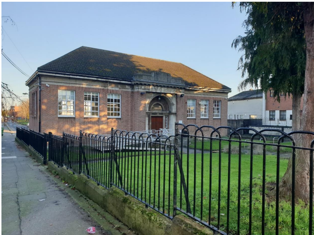
Library – Proposed Ballymun underpass to allow unimpeded passage from Blessington Street Park
